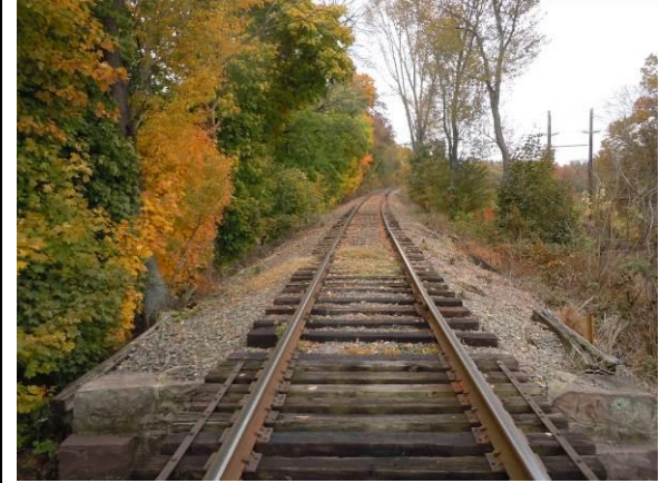
Surfacing projects is from the south abutment of Bridge 9.75 which spans the 3rd Neshanic Creek.
