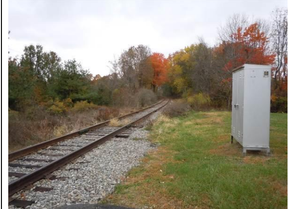
Everetts Road facing North.
