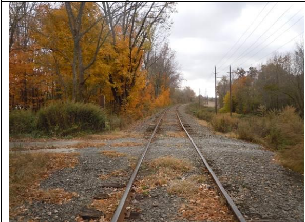
Private Crossing 8.54 facing South.
